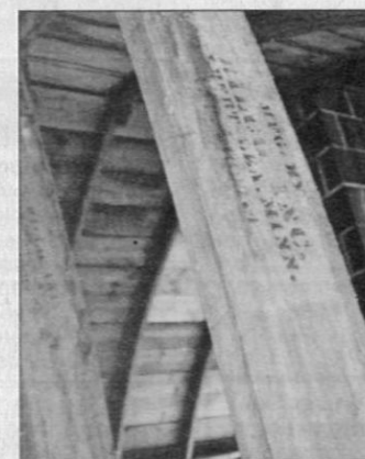
Laminated arch trusses by Rilco give the barn its historic heft.
